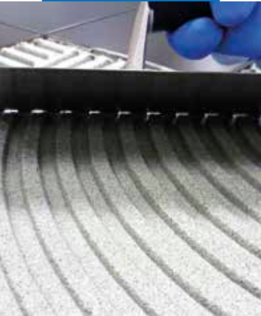
Installing ceramic tiles
